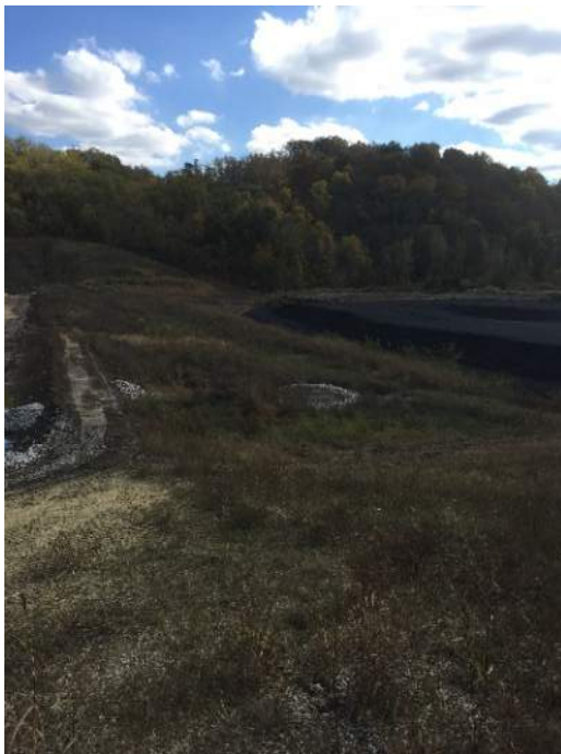
Photo 40 Sediment trap of pond at west end of landfill.
